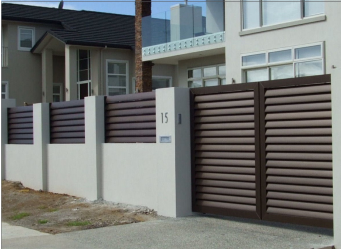
Vehicle access Gate, twin Hinged with Louvre infill. Fence, between nib walls with same infill
