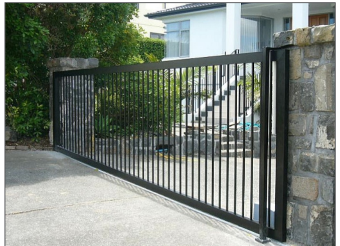
Vehicle access Gate, Sliding with Baluster infill.
